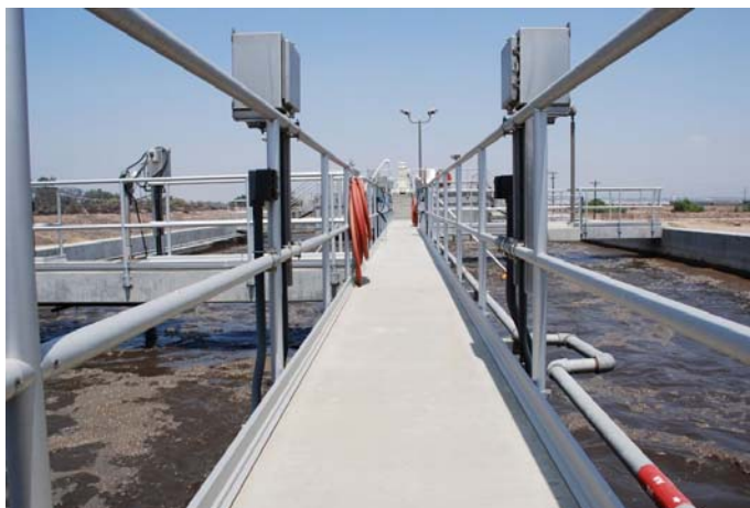
WMWD March WWTP
