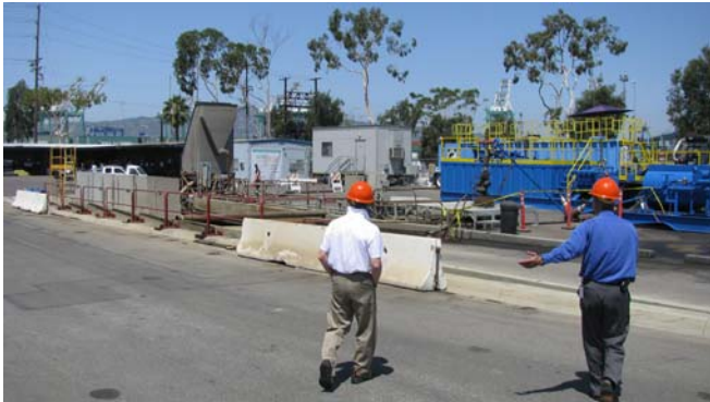
Omar Moghaddam leading tour of the Terminal Island Renewable Energy project located at the Terminal Island WTP.
