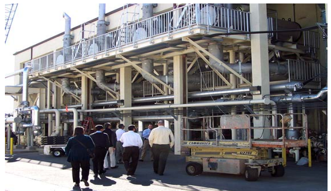
Encina WA’s newly constructed cogeneration facility.
